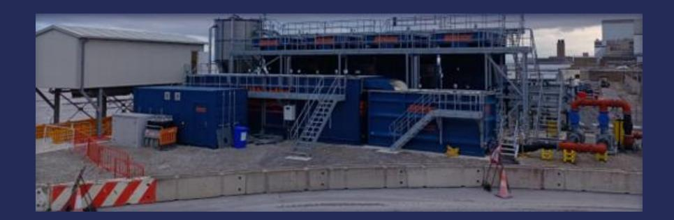
We planned for the commissioning of the Train B advanced surface water treatment plant to remove suspended solids from the surface water treatment process. We have been also been planning the commissioning of Mechanical Biological Bioreactor (MBBR) unit equipment which will enhance the biological treatment of the wastewater at our sewage treatment plant and the Dissolved Air Flotation unit which will help to remove solids from the treatment process.
