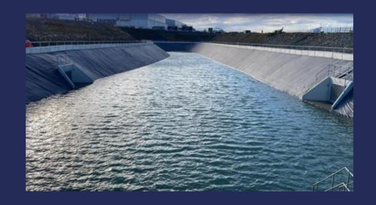
19,520 m3 of surface water taken from our Water Management Zone attenuation ponds was collected by tractor bowsers and re-used on Hinkley Point C site for dust suppression to improve and control the local air quality.
