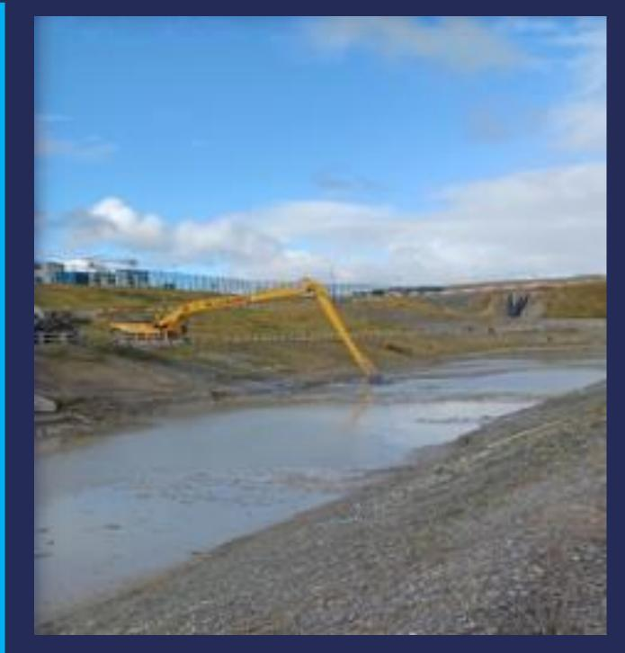
6,283m³ (133 tanker loads) of silt was removed from three of our Water Management Zone treatment ponds which is the equivalent of 78,500 baths full of liquid.
